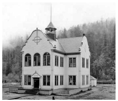
Aside from the remarkable choice of facade and trim, another interesting design feature was the tee shape, with the entrance at the foot of the tee. Later diagrams indicate the first room was a classroom, without an apparent hall to the rest of the building. Difficult to see in most images we have of this school is the exterior walls were milled tongue in groove boards like Skykomish Hotel and Maloney's Store.
